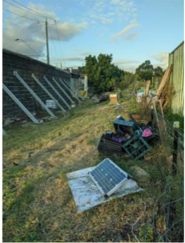
Photo 7: Swale area on northern side of site, which requires frequent brush cutting
